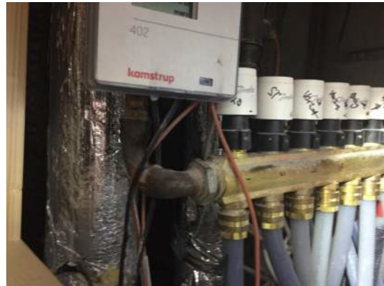
Figure 7. (a) The picture of flat substation taken by thermographic camera when the setpoint in one room was increased, and (b) The marks on actuator telling the name of the controlled room
