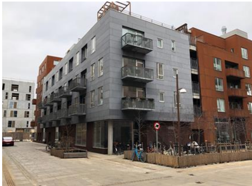
Figure 1: Havnehuset, located at Aarhusgade 140.
