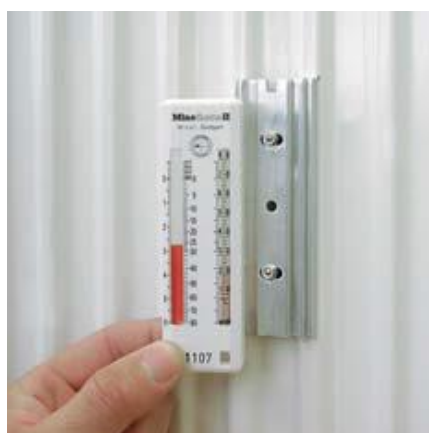
Figure 23. Capillary heat cost allocator
