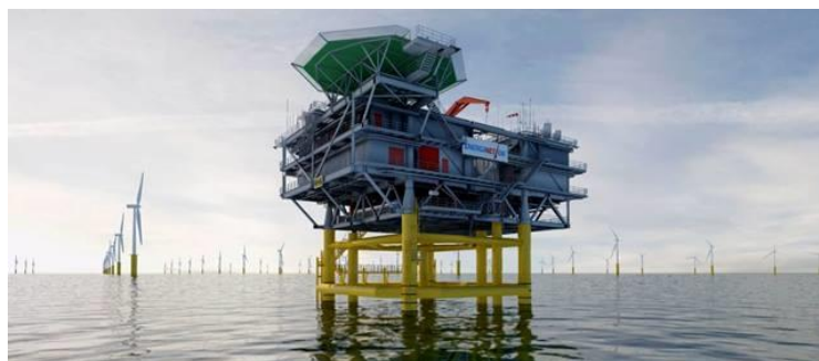
Figure 1 Offshore substation at Anholt windfarm [10]
