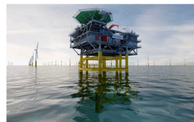
Fig. 2. Offshore substation at Anholt windfarm.
