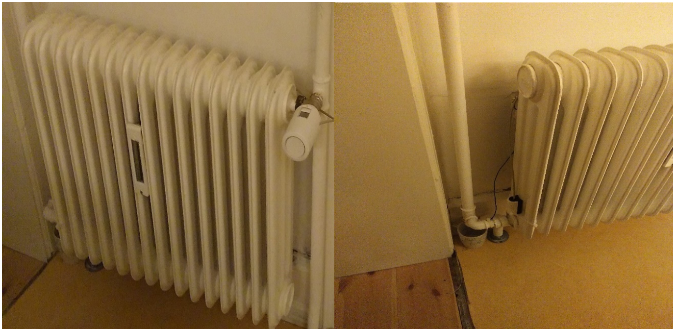
Figure 5. Pictures of the prototype thermostat and return temperature sensor and how they were installed on the supply ( left ) and on the side of the radiator ( right ) in the test buildings.
