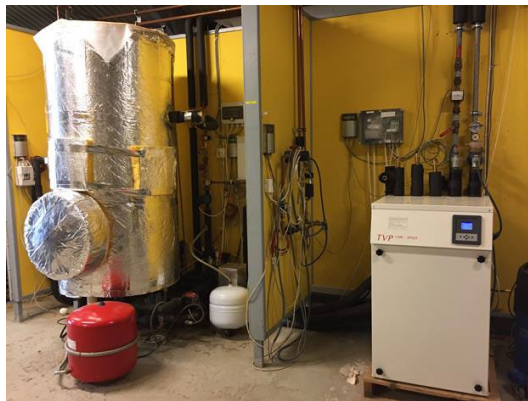
Fig.2 An overview of the SGHP system with measurement and controller sensors locations
