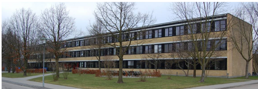
Fig. 1. Building 118 of the DTU campus at Kgs. Lyngby, Denmark.
