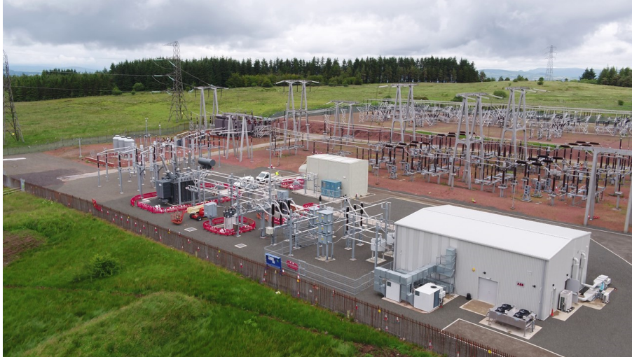
Figur 1.4: 140 MVA H-SC installed as a field trial of Phoenix project at Neilston, Scotland [3]
