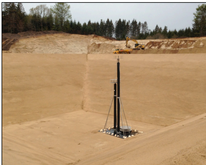
Fig. 4. Diffuser installation in Dronninglund [27].
