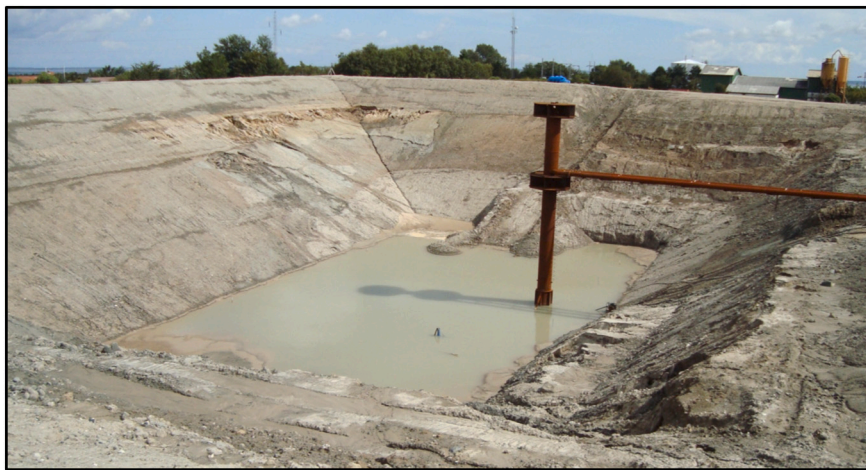
Fig. 2. Diffuser installation in Marstal [22].
