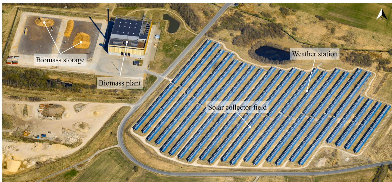
Fig. 2. Aerial view of the solar collector field, biomass plant, and outdoor biomass storage area belonging to the Brønderslev hybrid plant. Image source: the Danish Agency for Data Supply and Efficiency.
