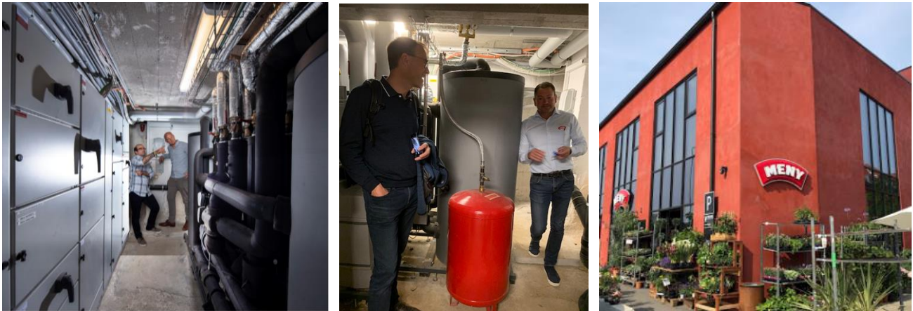
Figure 1: Heat is recovered from a supermarket refrigeration system to the local district heating grid in Nordhavn, Copenhagen.
