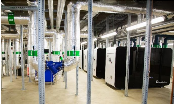
Figure 2: An Energy Machines installation. Heat pumps are located on the right. Sensors are placed inside the boxes.
