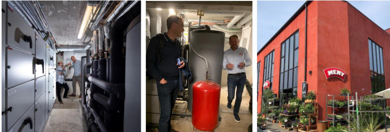
Figure 13. Heat is recovered from a supermarket refrigeration system to the local district heating grid in Copenhagen.
