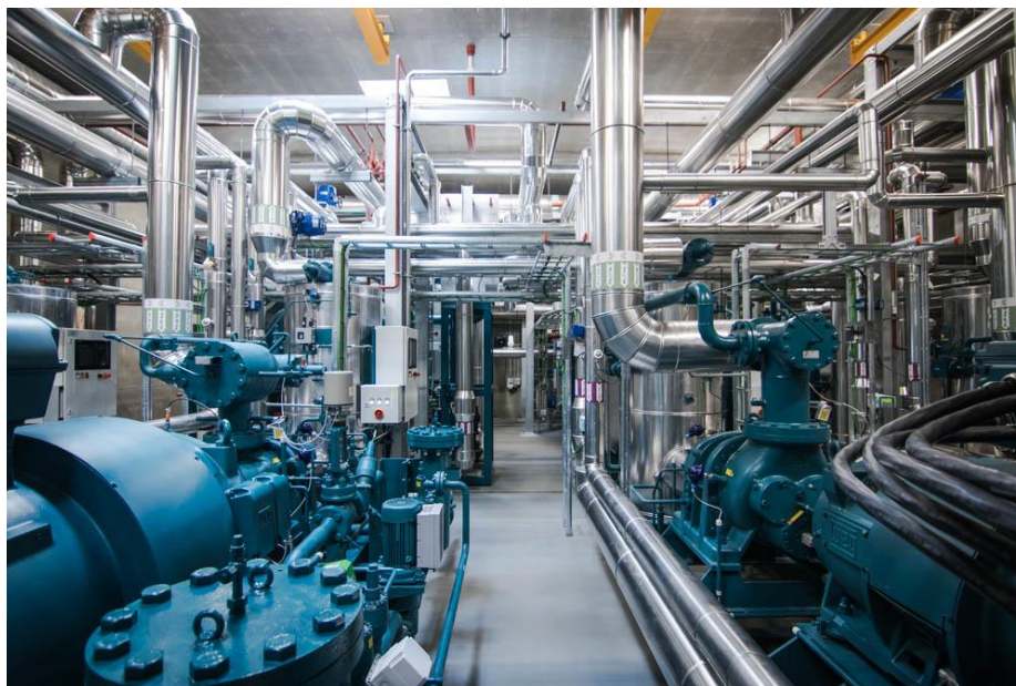
Figure 1: 5 MW thermal heat pump system for district heating in Copenhagen [Source: HOFOR].
