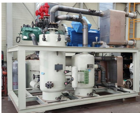
Heat Pump Unit (before casing)
