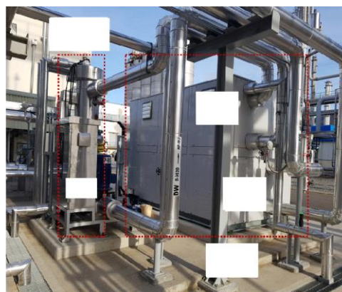
Figure 4-65 Field test and evaluation of steam heat pump at LG Chem.
