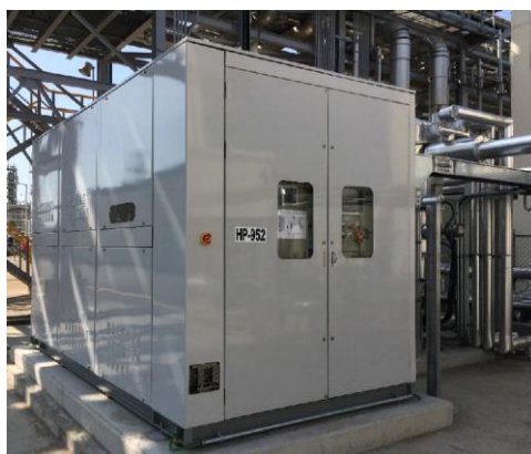
Figure 4-65 Field test and evaluation of steam heat pump at LG Chem.
