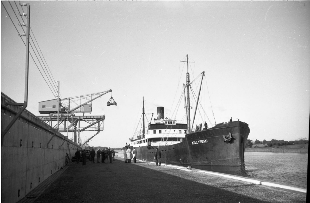
Image 3. The first coal for the new energy plant located next to Odense Canal arriving in the cargo ship Myllykoski in 1952. In the first years of operation, one collier would arrive with enough fuel for the entire winter season. Source: Fyens Stiftstidendes pressefotosamling, Odense Stadsarkiv.
