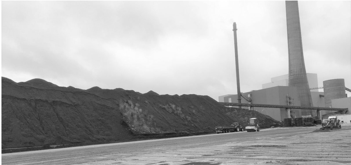
Image 2. The last piles of coal to be used for district heating in Odense before it is phased out as fuel.
