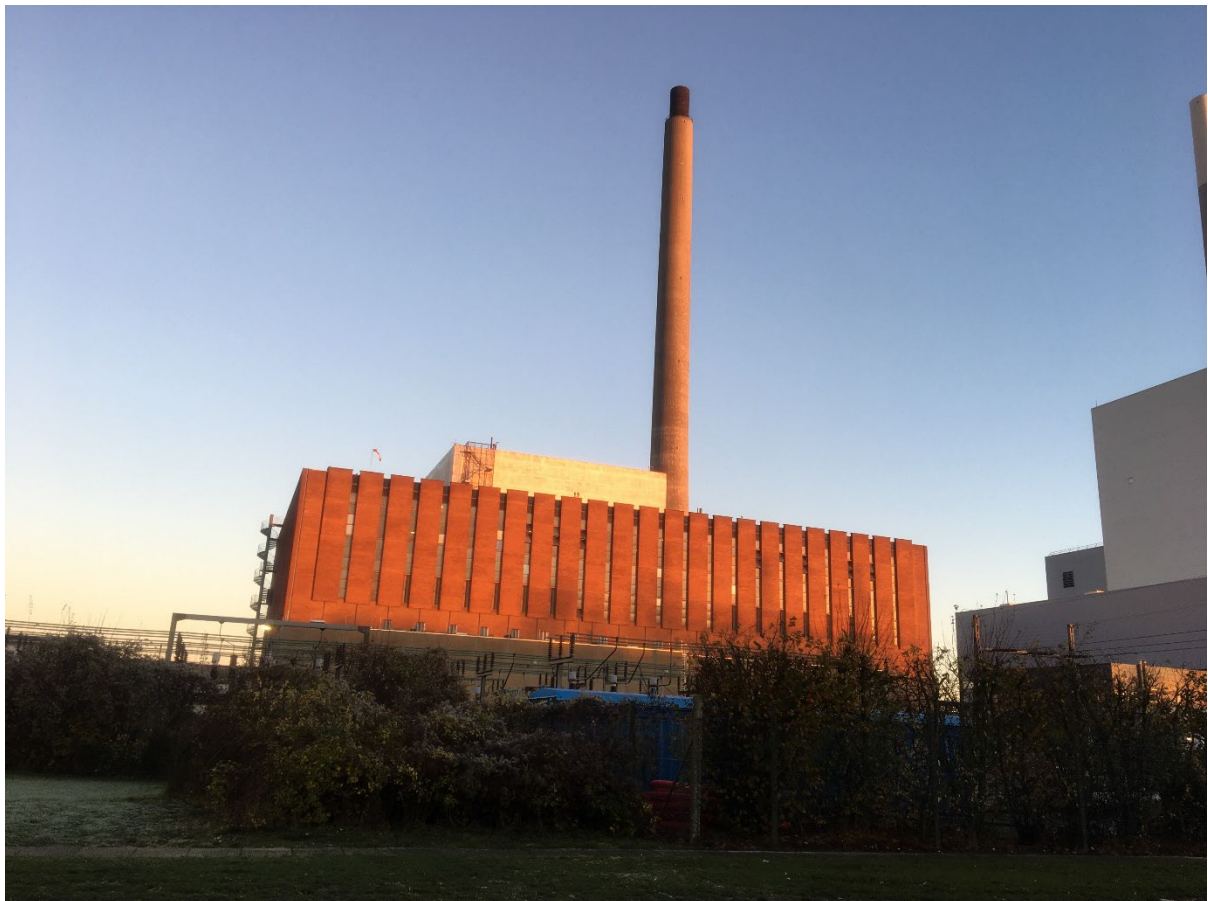
Image 1. A building hosting a coal boiler in Odense on a cold day in 2020. Photo by the author.
