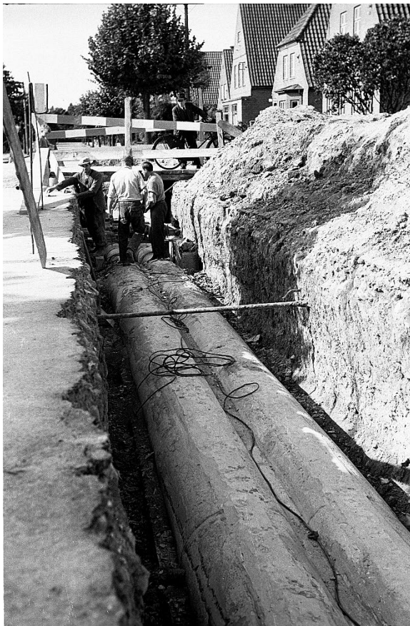
Image 4. New pipes are constructed to connect more areas of Odense to the large new energy plant in 1952 – here at Ærøgade 22. Source: Fyens Stiftstidendes pressefotosamling, Odense Stadsarkiv.
