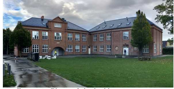
Figure 1: Photo of the building in question.
