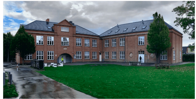
Fig. 1. A photograph of the building site.
