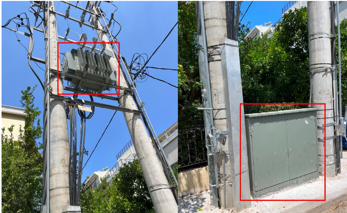
Figure 3.2: Outdoor Secondary Substation with 5 LV feeders. Transformer (left) and LV Combiner Box (right)
