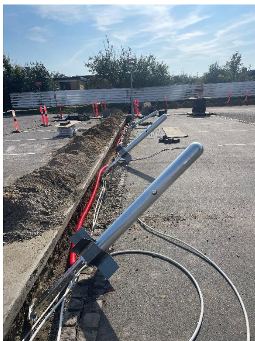
Figure 8: Cables are in the ground and poles are ready to be fixed in the ground.
