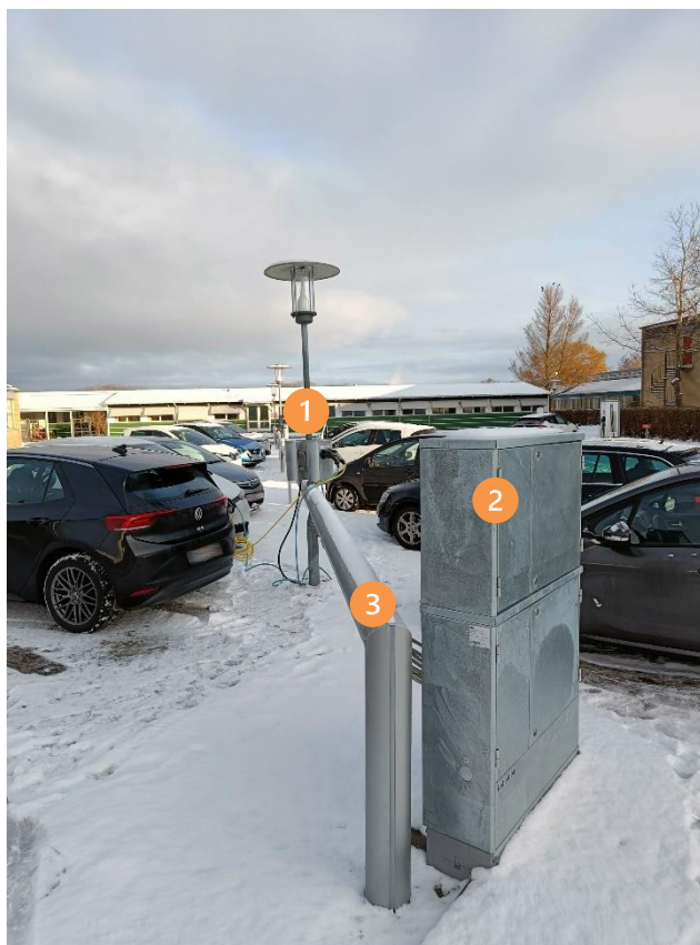
Figure 2: Charging infrastructure in Risø. 1) Chargers; 2) PCC cabinet for all EVSE connections; 3) Cable tube for connecting chargers to PCC cabinet.
