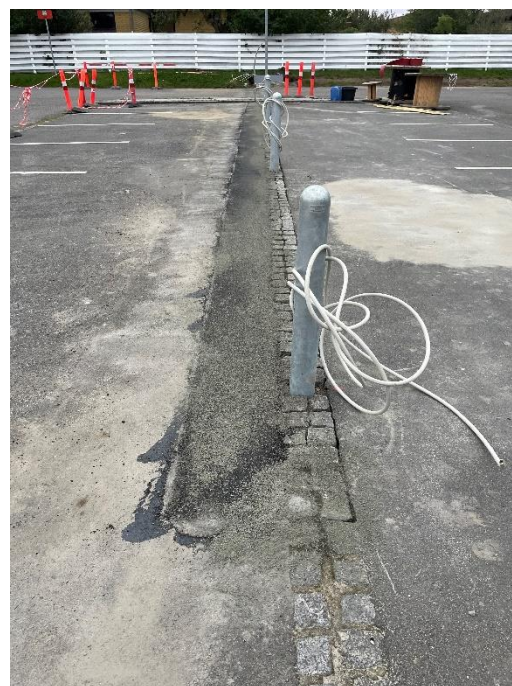
Figure 9: Poles are ready for installation of chargers.
