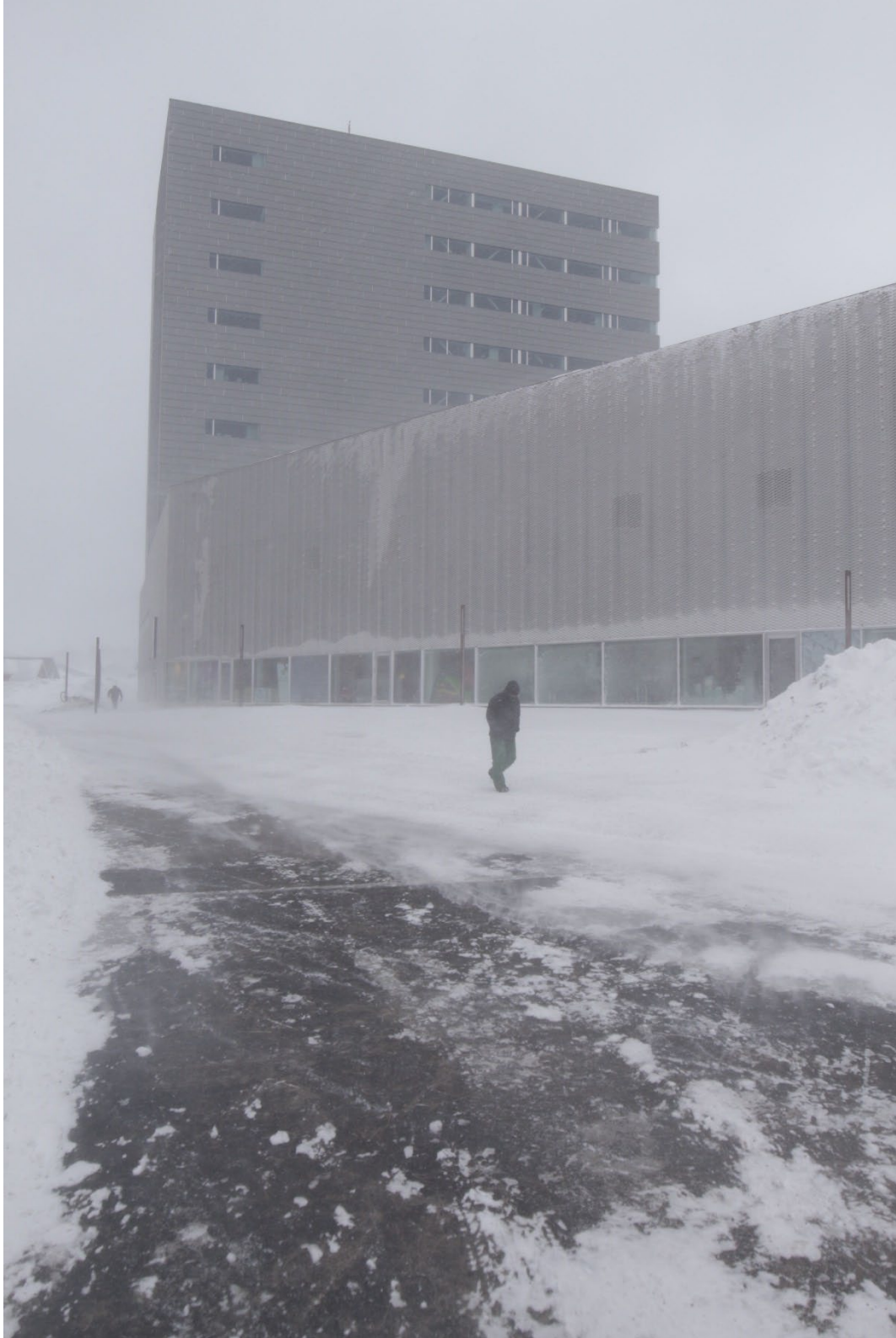
Figure 3 Nuuk Center when snowdrift has a large impact on the structure of the building façade. Snow particles with strong adhesion deposit at metal grid façade. People walking by struggle to pass the high-rise tower at high velocities.
