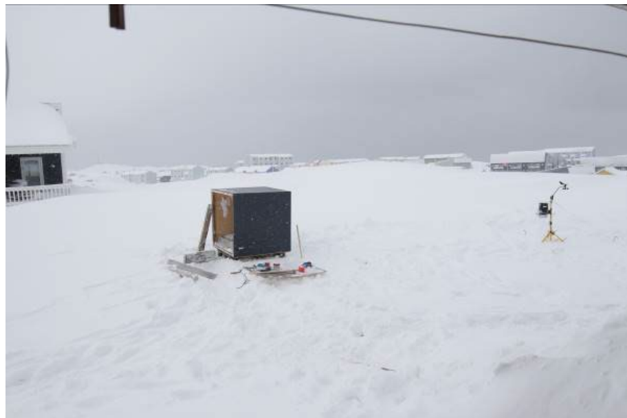
Figure 31 Installation and assembly of the Nuuk Cube Field Experiment on the outskirts of Nuuk City in March 2017.
