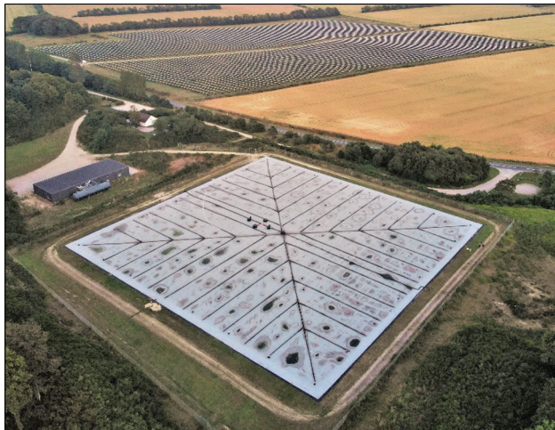
Fig. 1. Aerial view of the PTES and solar collector field in Dronninglund.
