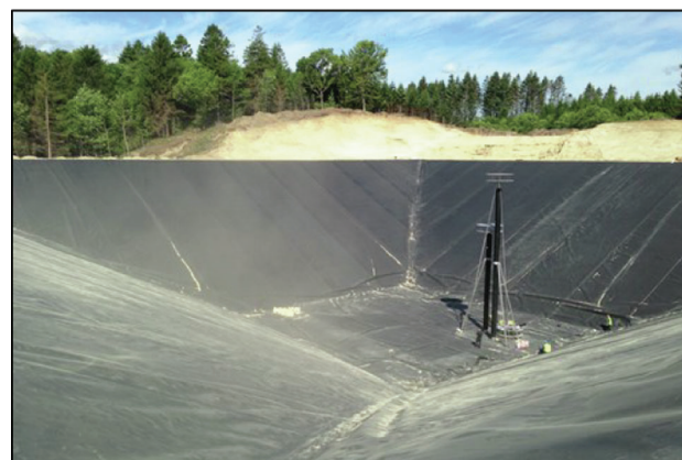
Fig. 5. Installation of the bottom liner of the Dronninglund PTES (PlanEnergi).
