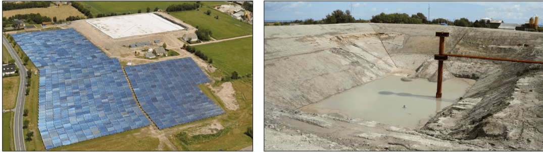
Figure 2.1: Aerial photo from 2013 (left) and diffuser installation in the PTES in Marstal (right) (PlanEnergi, 2013).
