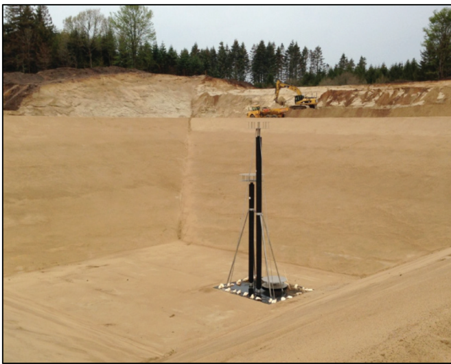
Fig. 4. Diffuser installation in Dronninglund [27].
