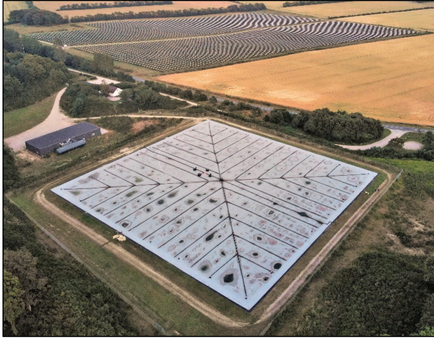
Fig. 3. Aerial photo of the PTES in Dronninglund in 2019.
