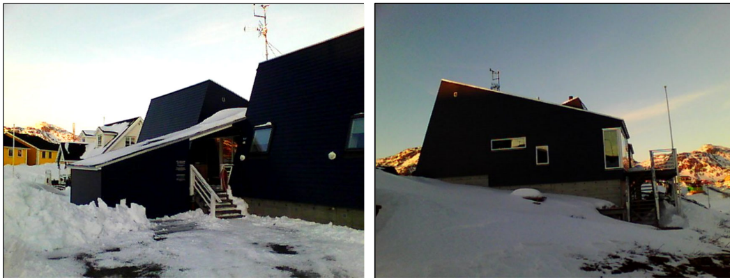
Figure 2.9. Photos of the Low Energy House in Sisimiut (March 2021).
