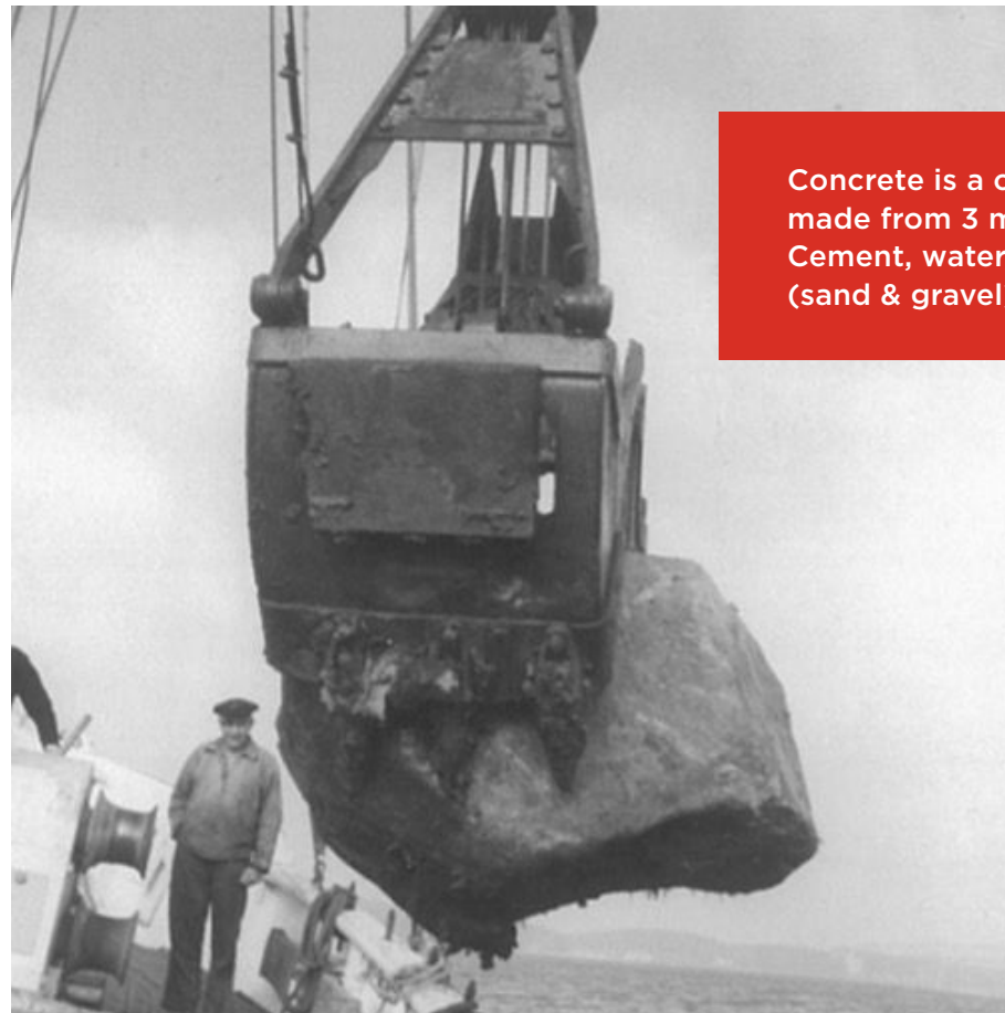
↑ Figure 2: Stone fishing conducted with a mechanical crane.
