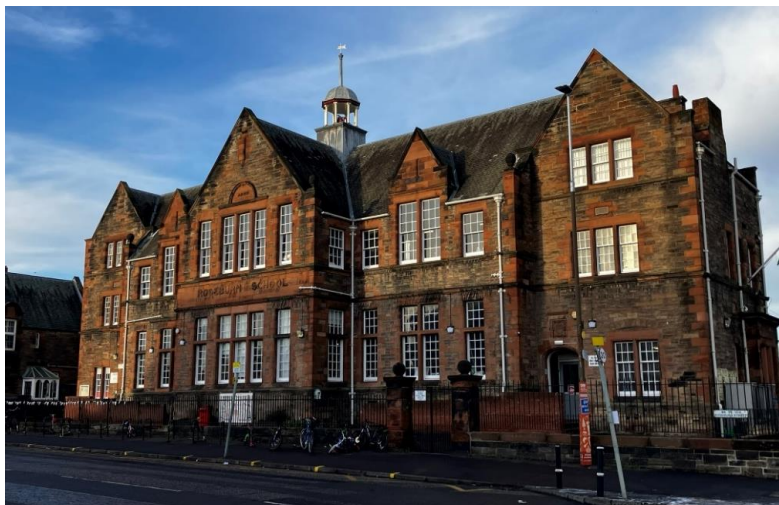
Photo 1: External view of the primary school. Main façade.
