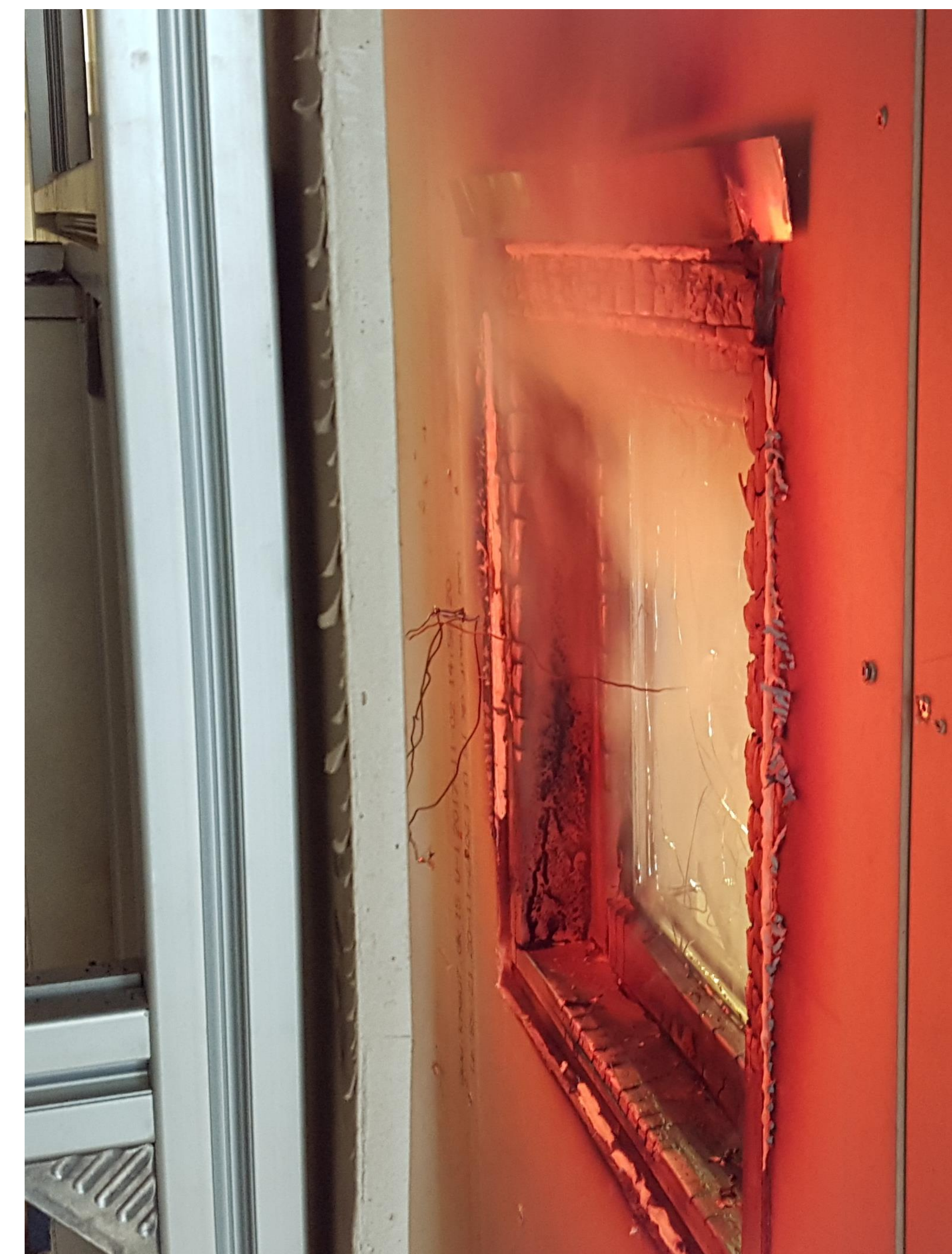
Fig. 3: Cracked glass and charring wood frame on exposed side. Photo by Nielsen [4].
