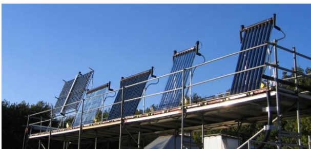
Fig. 8: The test facility at DTU Byg.
