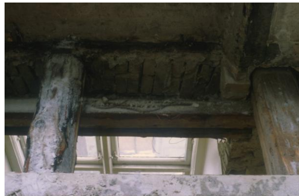
Fig. 2: Support of beams in the wall (danskbyggeskik.dk).
