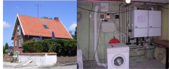
Left: Demonstration house before installation of the solar heating system. Right: Non condensing natural gas boiler and separate hot water tank.
