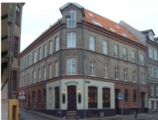
Fig. 1: Multi-storey building in masonry, Danmarksgade, Aalborg (arks.dk).
