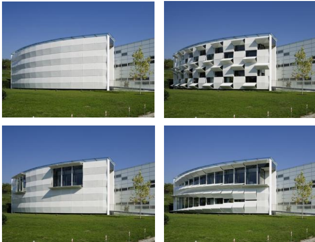
Fig. 4: The Showroom for Kiefer Technic shows an example of a dynamic façade and its possible influence on the over-all aesthetic appearance.
