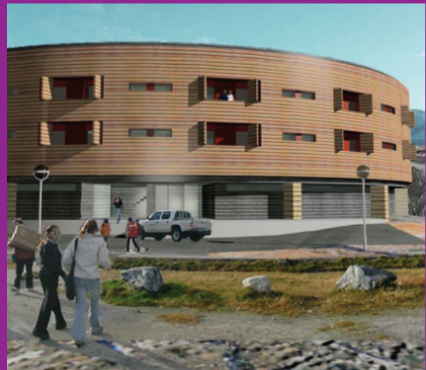
A new highly energy-efficient dormitory building currently being constructed in extreme climate conditions at Sisimiut, Greenland. Illustration: tnt-nuuk a/s
