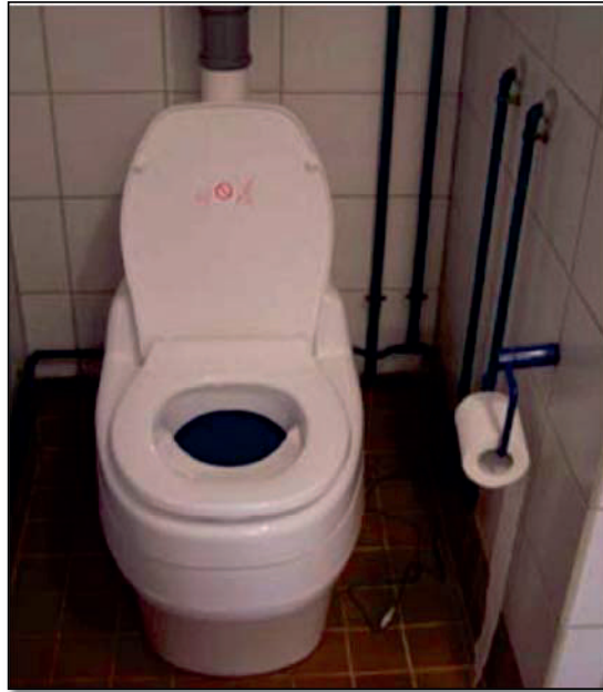
Figure 2.4. A urine separating composting toilet (Villa 9010) which was tested in a single-home residence in Sisimiut, West Greenland (Picture: Ragnhildur Gunnarsdóttir)
