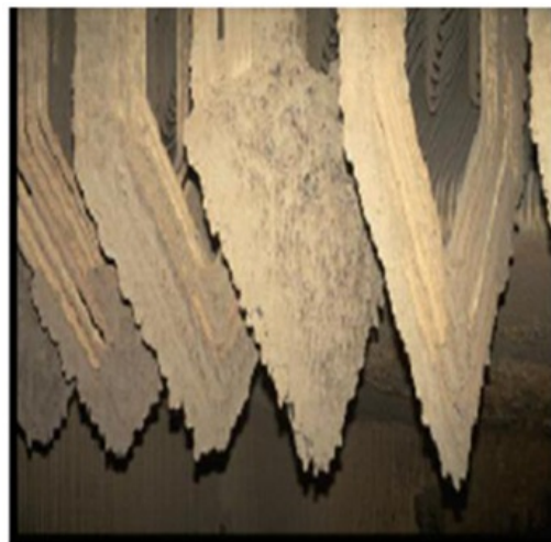
Figure 2.12: Ash deposition on the superheaters during straw and coal co-firing [2].
