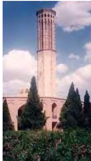
An octagon wind tower in Yazd
