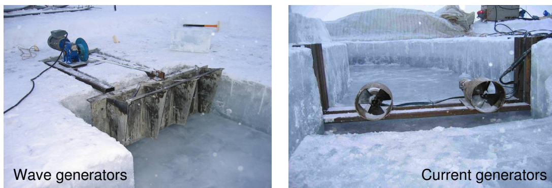
Figure 3 Wave generator (left) and current propellers (right).
