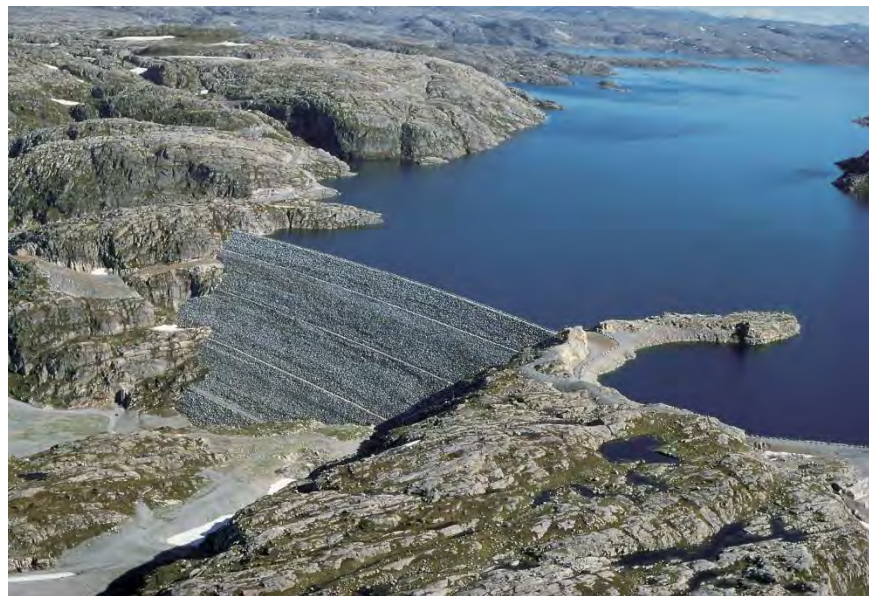
Figure 2.3. Oddatjørndammen in Rogaland, Norway's highest rock-filled dam (142 m) and the Blåsjø reservoir, which form part of the Ulla-Førre hydropower complex.
