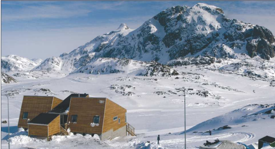
Figure 1: Picture of the low-energy house in Sisimiut.
