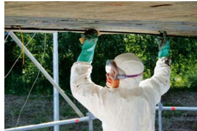
Placing the high quality carbon fibre rods in the pre-sawed slots helped the bridge to resist a load increase from 2 MN to 12 MN before failure
