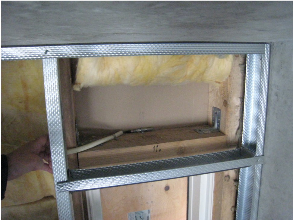
Fig. 36. Vaisala sensors, module line 3-4, DTU11 from inside, close-up 2
