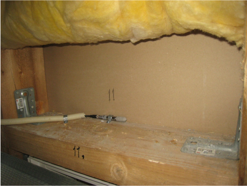
Fig. 35. Vaisala sensors, module line 3-4, DTU11 from inside, close-up
