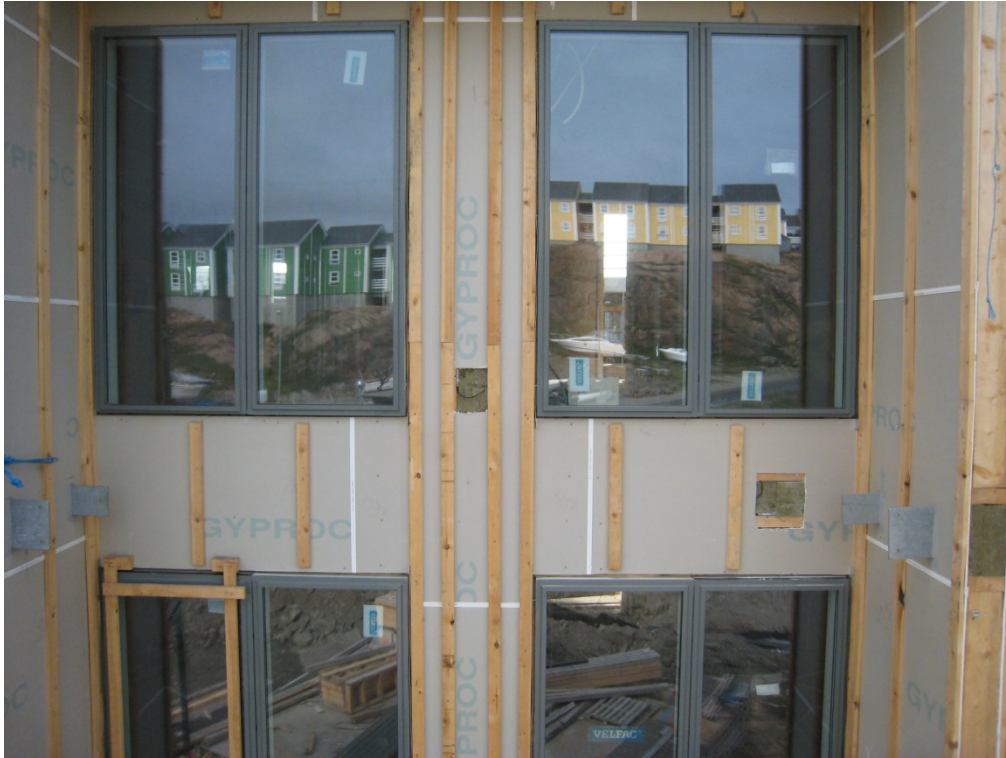
Fig. 17. Vaisala sensors, module line 3-4, DTU3 and DTU8 from outside
