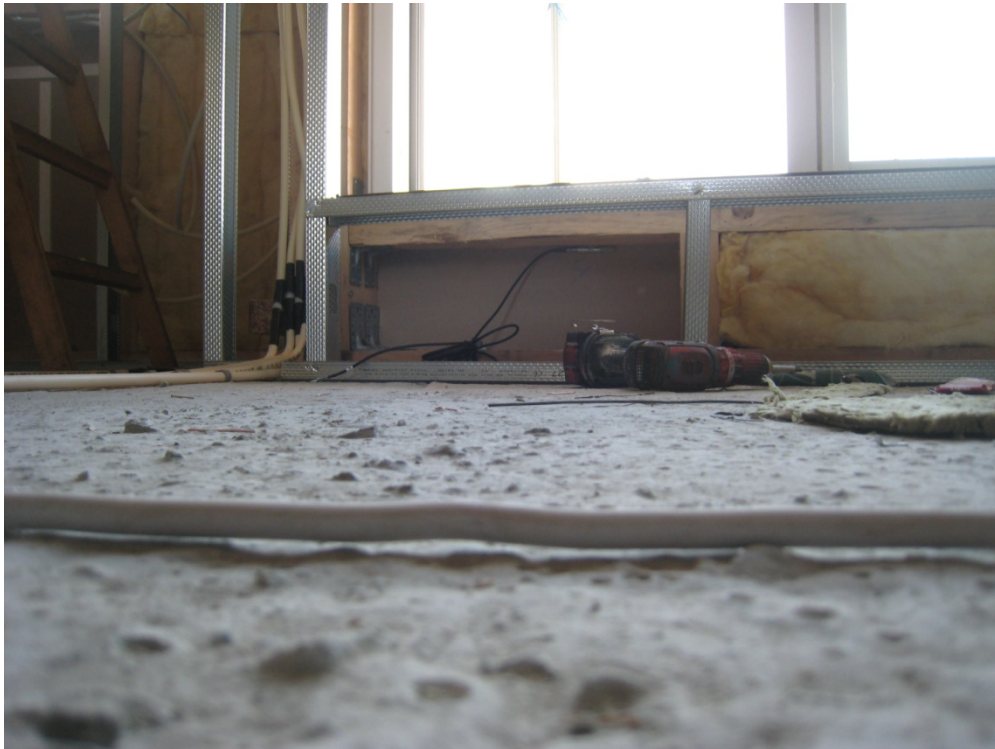
Fig. 30. Vaisala sensors, module line 3-4, DTU9 from inside
