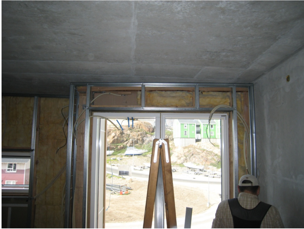
Fig. 23. Vaisala sensors, module line 3-4, DTU5 and DTU6 from inside
