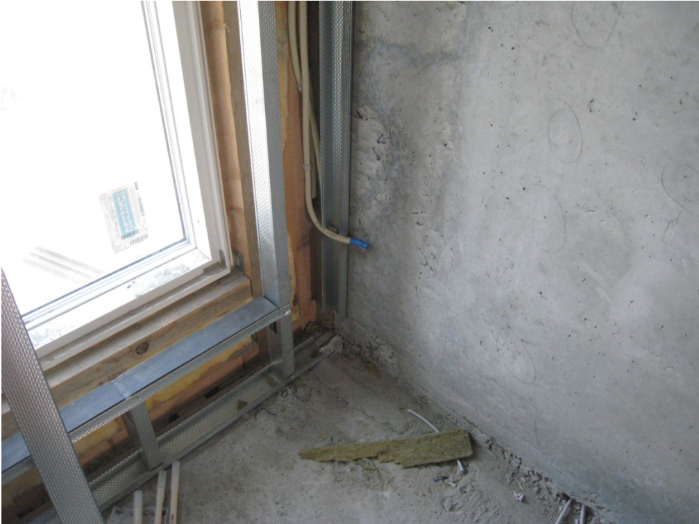
Fig. 14. Vaisala sensors, module line 3-4, DTU1 and DTU2, from inside
