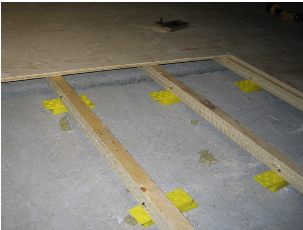
Figure 6.20 Floor construction. A wooden floor on rafts is used. A plywood plate of 15mm is used as the floor covering. In the room, a 6mm parquet floor is placed on top of the plywood plate.
