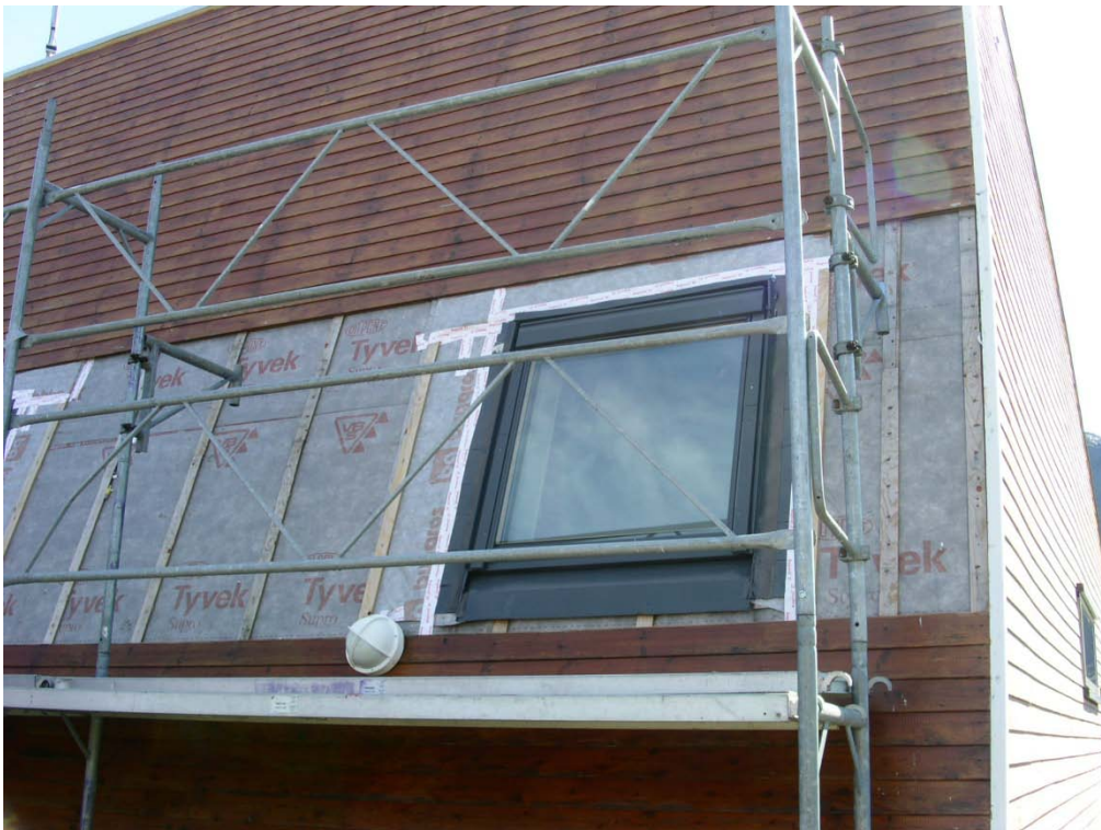
Improving the air tightness (summer 2010)
