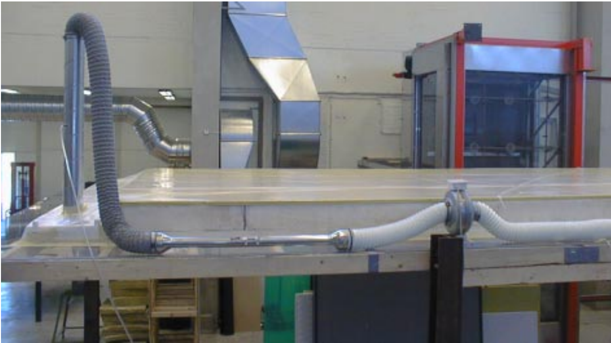
Figure 10.22 Vertical duct at the air outlet, the steel pipe for measuring the air flow and the ventilator
