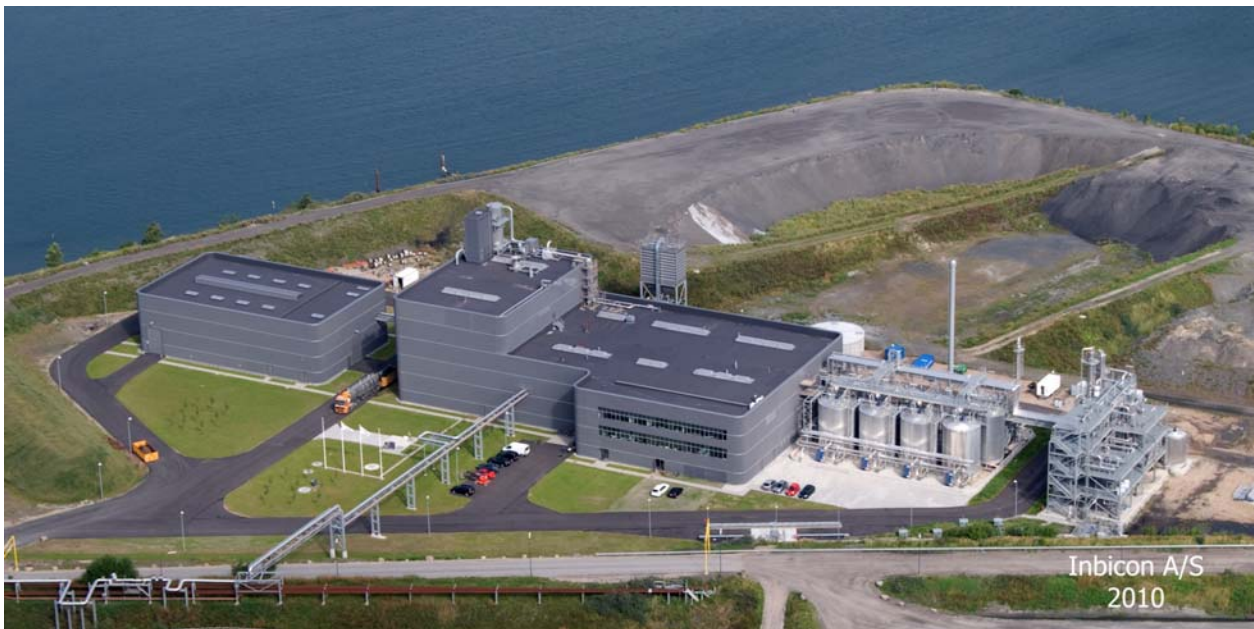
Figure 3: INBICON in Kalundborg - the world's largest 2G bioethanol plant. Produces bioethanol, molasse and lignin pellets from straw - capacity to convert 100 tonnes straw per day.
