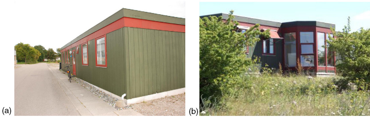
Fig. 3. (a) The north facade and (b) is the south facade of the building.
