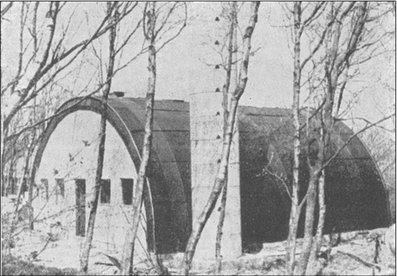
F.C. Becker's "Almost-Heat-Tight" house, that he built in North Zealand on his own money. The tower in front was designed for a windmill.
