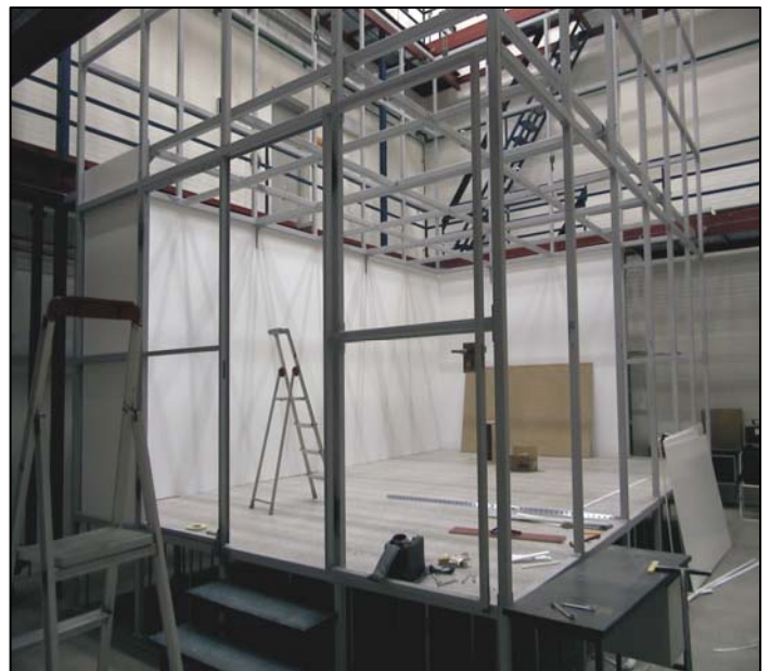
Climate chambers for study of airflow in rooms. The size can be changed and it can be divided into several chambers.
