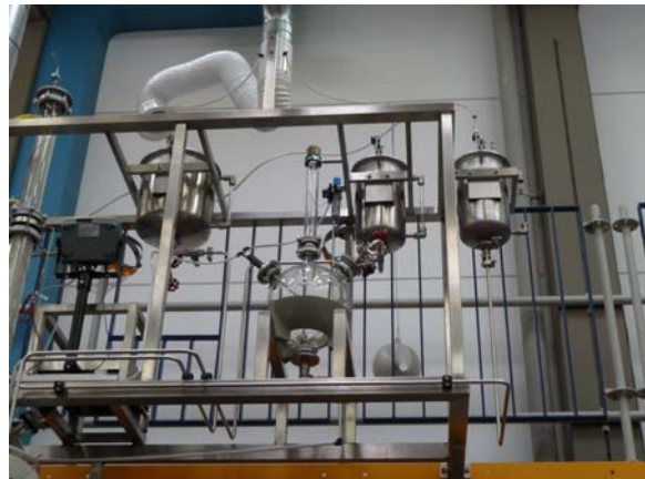
A pilot plant for enzymatic biodiesel production (feeding tank part)
