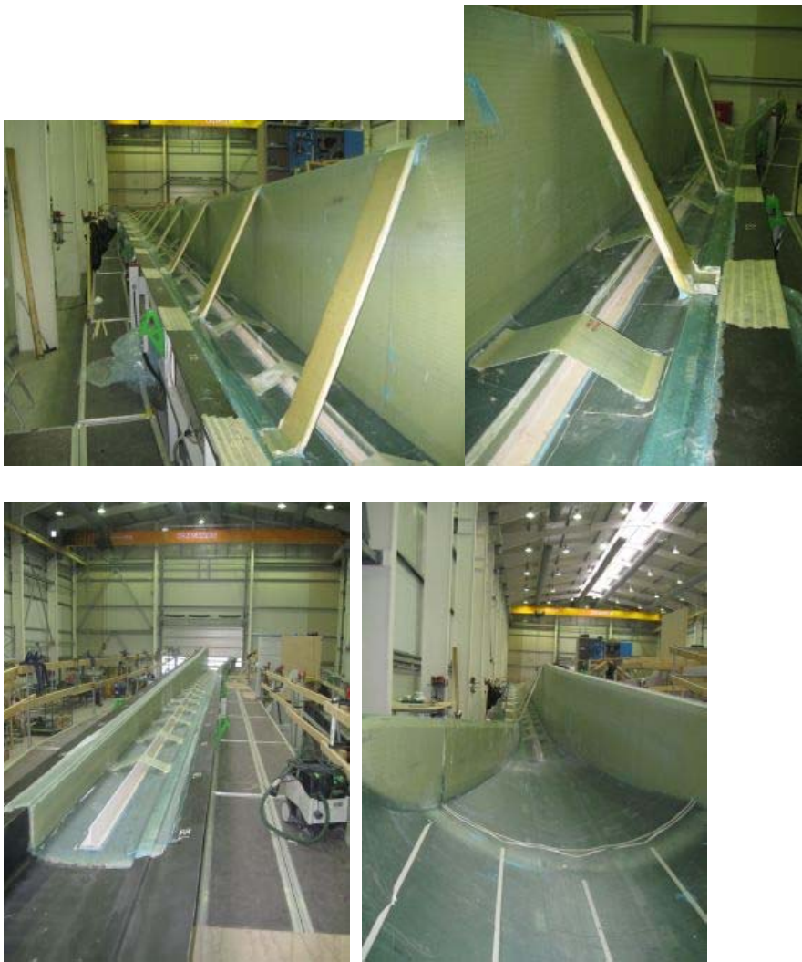
Figure 47: Photos of the cured parts with the reinforcements installed
