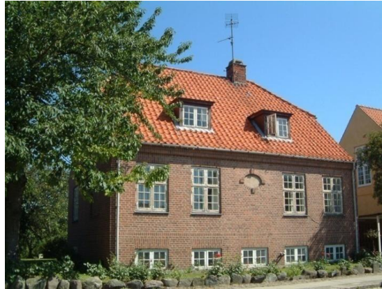
Figure 4. Typical old master builder houses built in 1927, having a full basement.
