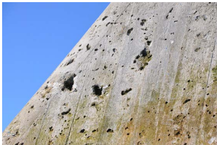
Figure 3 – Deep holes into the concrete surface.
