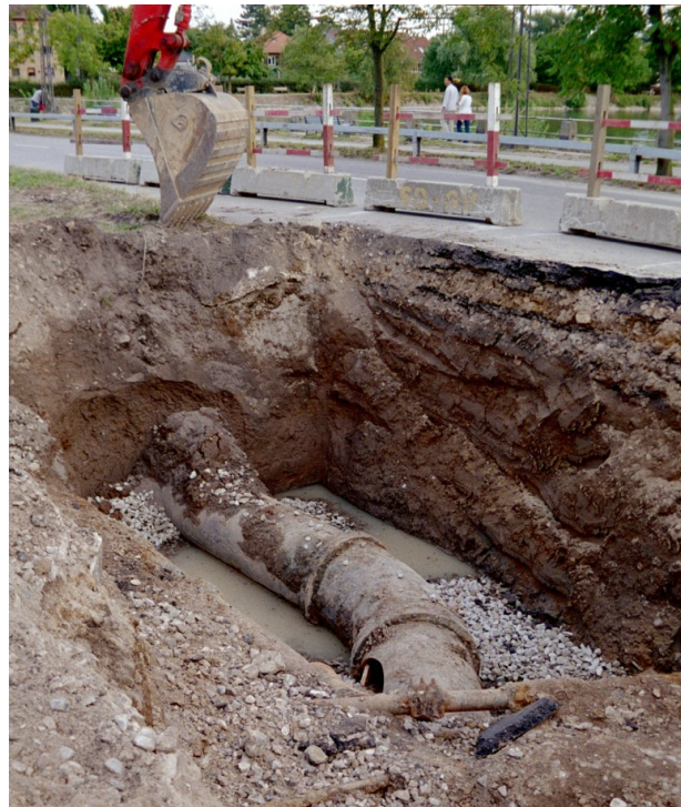
Figure 3-3. Burst pipe awaiting repair. Water is not properly drained from the hole. Photo: H.-J. Albrechtsen.
