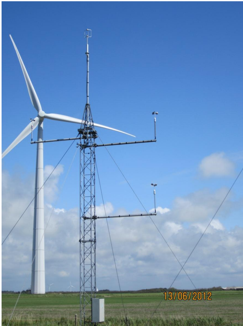
Figure 8 The mast for the reference sonic anemometer at the Høvsøre test station.
