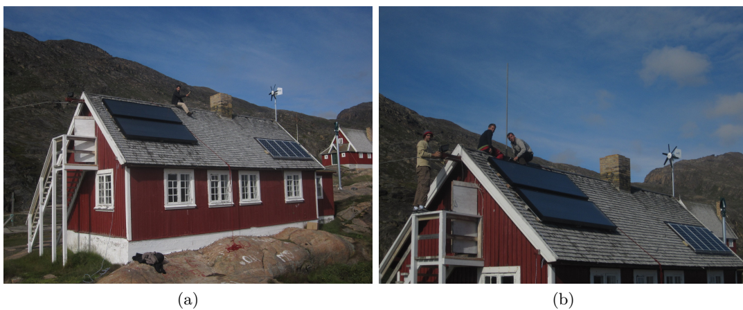
Figure 1.3: Mounting of a small mast on a roof at Assaqtuq.
