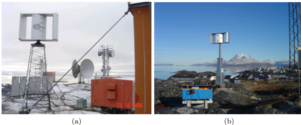
Figure 10.2: Examples of wind turbine used by Telegreenland. (a) VRE.3xxx, 3000VA - (b) VRE.007, 750VA
