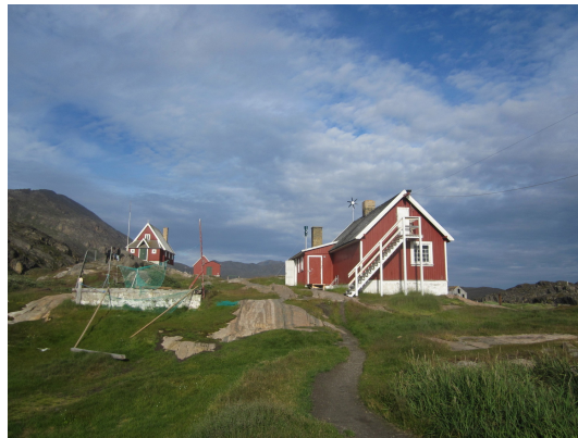
Figure 1.1: View of the best preserved houses of Assaqtuaq village
