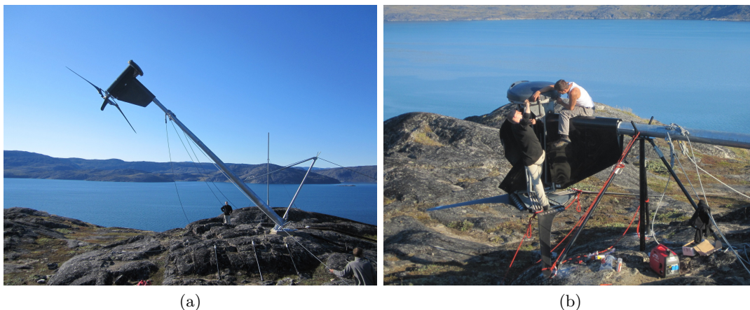
Figure 2.2: Work on the wind turbine at Sarfannguaq. (a) The turbine being put down - (b) Work on the brake pads inside the nacelle
