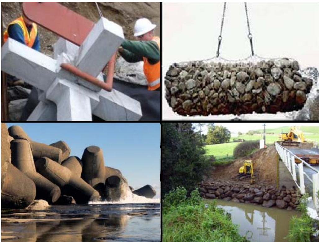
Figure 5-7 Examples for elements of different armour protection systems, top left: concrete A-jacks [ http://www.rocla.com.au/Popup_Gallery.php?id=458&category=ajacks ], top right: gabion sacks [ http://www.maccaferri-india.in/erosion-control-products.htm ], bottom left: tetrapods [ http://videohive.net/item/japan-tetrapods-2/1791603 ], bottom right: rock armour [ http://www.rintoulcivil.co.nz/projects5.php ].
