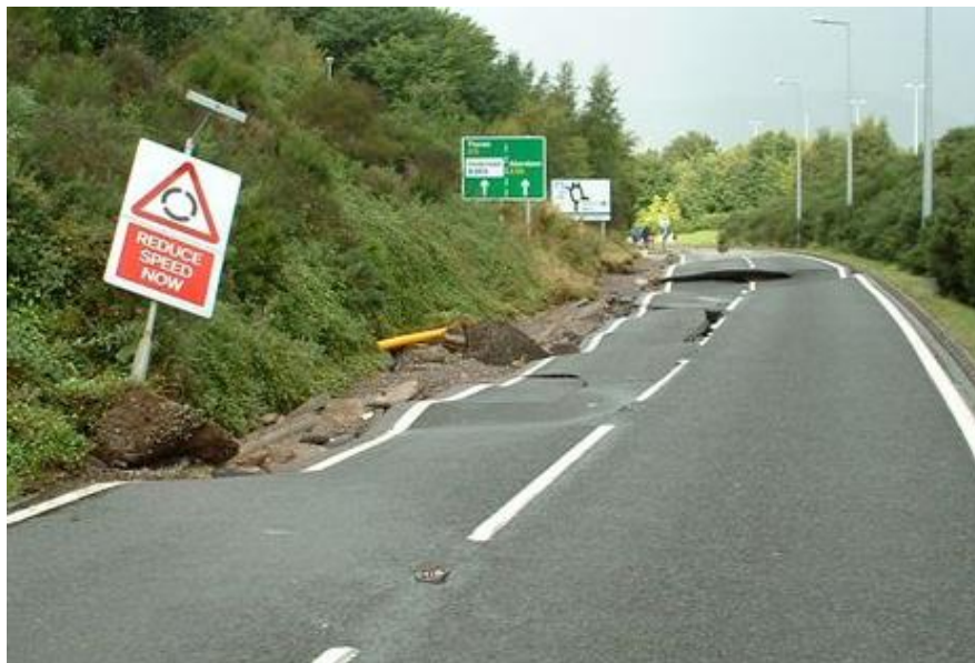
Figure 4-8 Damage to A9 Raigmore Slip Road, Inverness, 2002, following heavy rainfall. Photo by BEAR Scotland Ltd.
