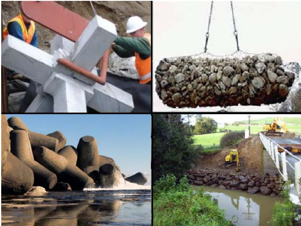
Figure 5-7 Examples for elements of different armour protection systems, top left: concrete A-jacks [ http://www.rocla.com.au/Popup_Gallery.php?id=458&category=ajacks ], top right: gabion sacks [ http://www.maccafferri-india.in/erosion-control-products.htm ], bottom left: tetrapods [ http://videohive.net/item/japan-tetrapods-2/1791603 ], bottom right: rock armour [ http://www.rintoulcivil.co.nz/projects5.php ].
