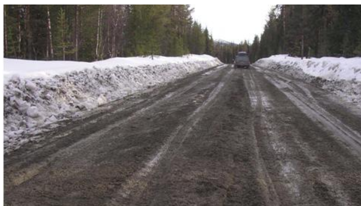
Figure 4-3 Frost damage on a gravel road in Raattama, Finland (photo J. Leskinen) [ www.tiehallinto.fi ]
