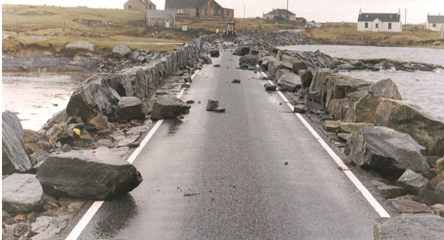
Figure 5-2 Damaged causeway in Scotland [ http://coastadapt.org/Outer-Isles/index.html ]
