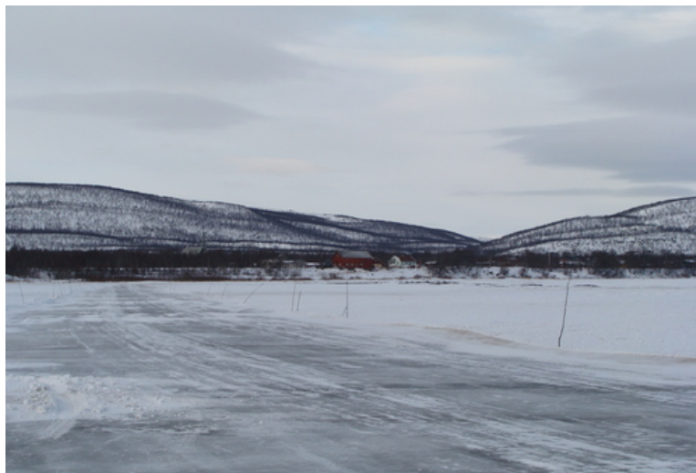
Figure 4-5 Ice road across Tana river towards Rustefjelbma [http://www.panoramio.com/photo/19664109]
