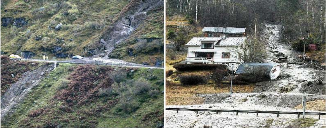
Figure 4-10 Examples for landslides from Scotland [ http://www.robedwards.com/2008/10/revealed-the-380-kilometres-of-road-most-at-risk-of-landslides.html ] and Norway [ http://www.aftenposten.no/english/article2402918.ece ].
