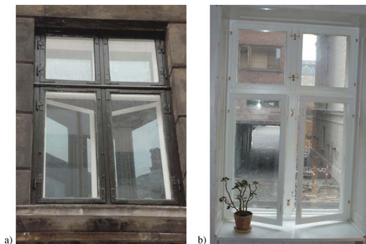
Fig. 4. Energy retrofitted 4-light Window 2 with a secondary frame seen from (a) exterior of building and (b) interior.
