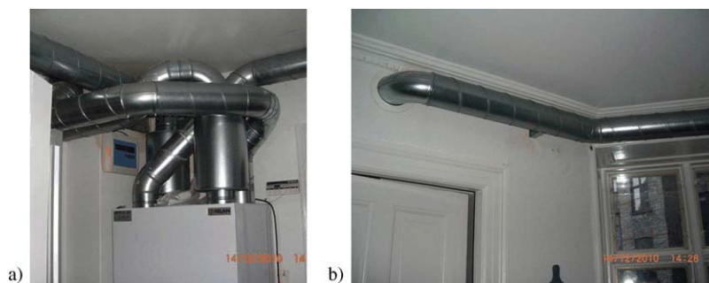
Fig. 10. Ventilation ducts in apartment. (a) Inlet and outlet from the air handling unit and (b) duct located in rooms.
