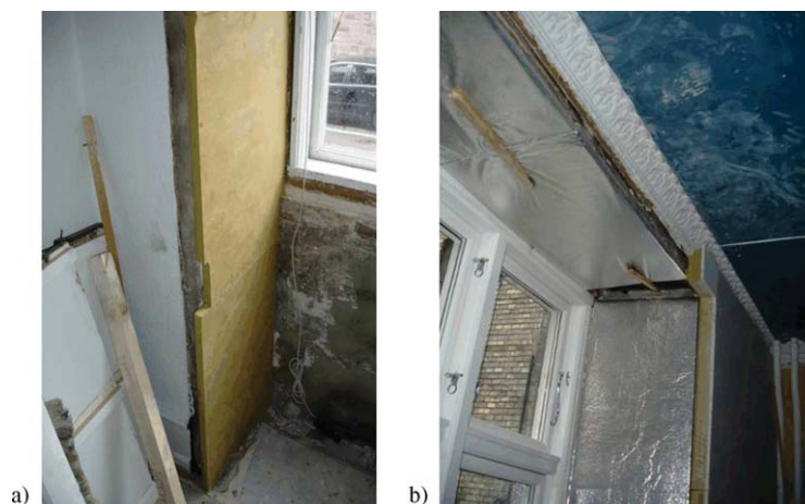
Fig. 7. Insulation applied in the window reveals where (a) is Aerowolle and (b) is Vacupor NT.
