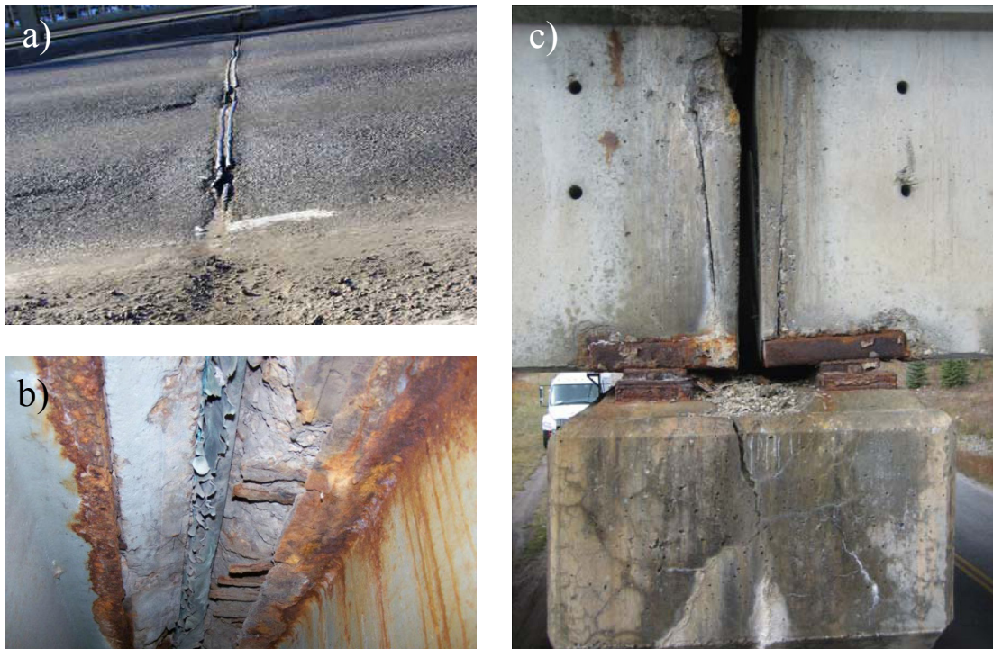
Figure 1-1 Examples of damage due to deterioration of expansion joints, a): in pavement on top of expansion joint (WSDOT, 2011), b): in severely corroded expansion joint seen from below (TCPI, 2012) and c): in girders and pier caps with highly corroded steel bearings (Ho and Lukashenko, 2011).
