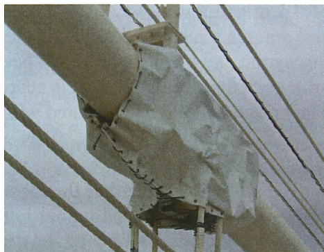
Figure 4: Cable band cover, reproduced from (Numata and Kitada, 2008).
