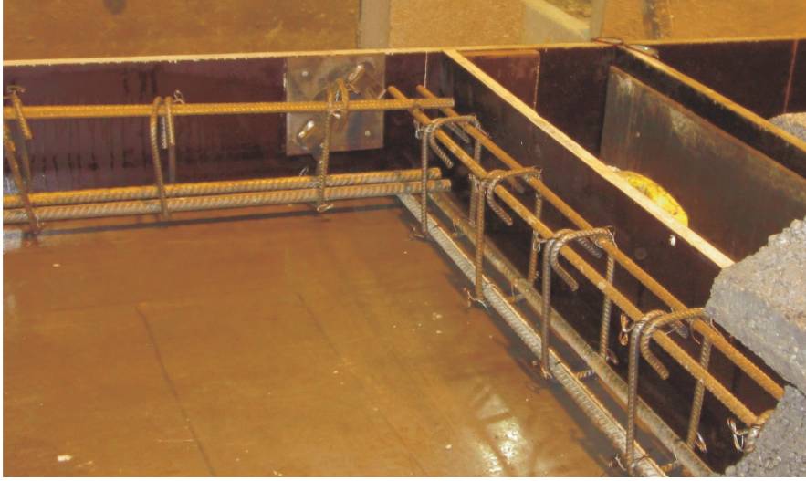
Figure 4: Beam reinforcement placed in order to create edge and end beams in a super-light element
